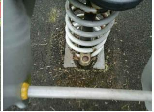
Finding: The U bolts clamping the spring are worn
