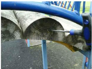
Finding: There is evidence of rot in the ends of the timber bridge sections
