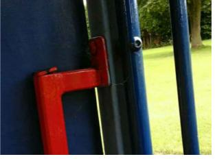
Finding: A number of fixing(s) have worked loose Action: Secure all loose fixings
