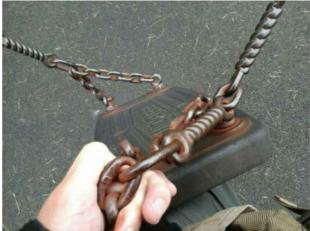
Finding: The chain links are worn in excess of 40%
