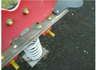
Finding: The Handgrips/Footrests rotate and may cause an unexpected movement for the user
