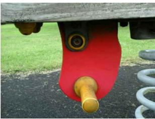
Finding: There is/are bolt cap covers missing or damaged on the item
