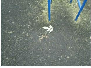
The safety surface under or around this unit has been damaged Monitor for any further deterioration and repair as required Finding: Action:
